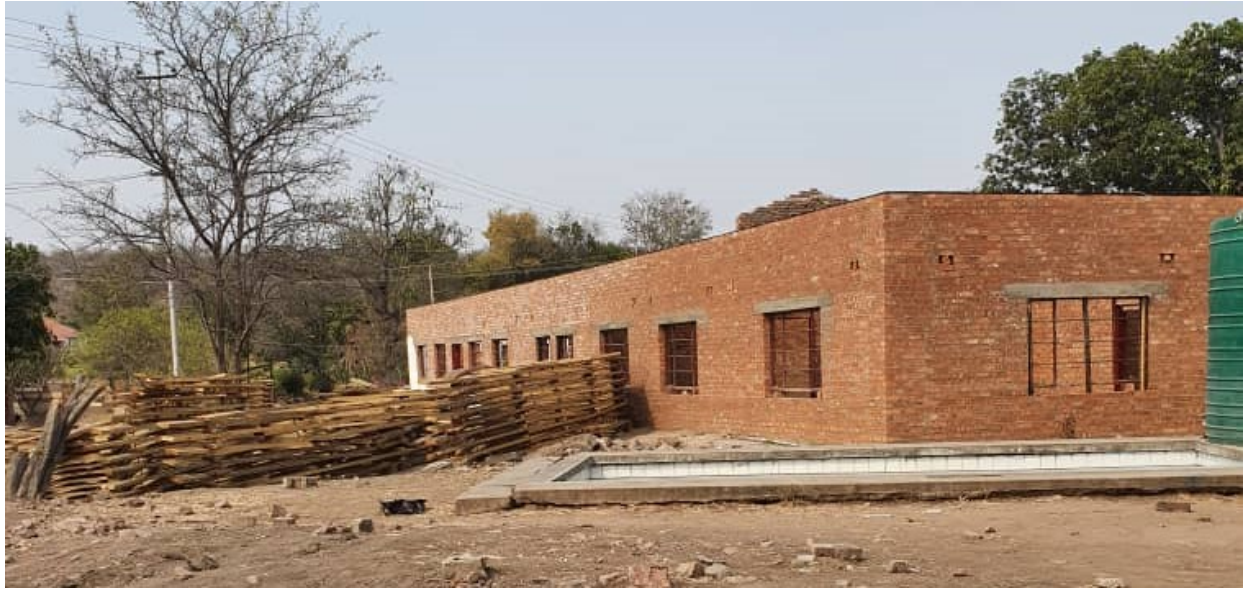
The library, computer laboratories and tutorial rooms at roof level.
