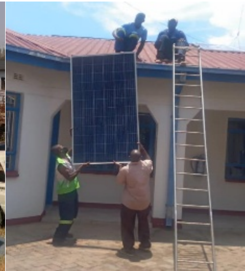
Solar panels being mounted at Masvingo Regional Campus
